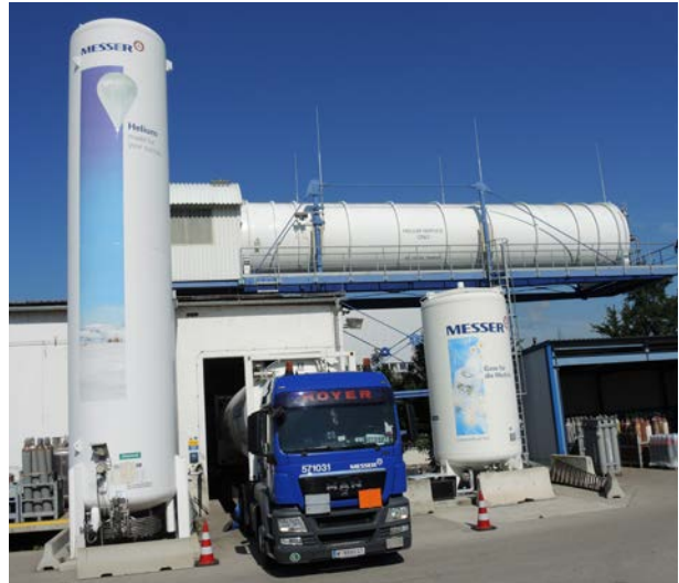
120,000 l horizontal tank container for liquid helium
